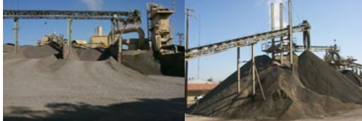
Stockpile and Conveyor System
